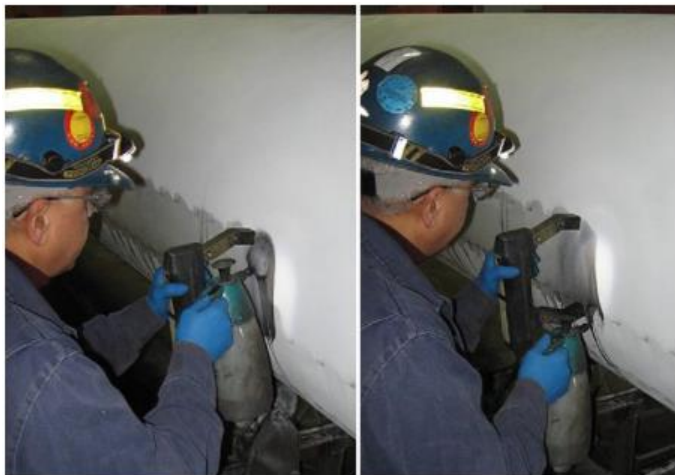
Figure 87. Magnetic Particle Testing of a Pipeline
