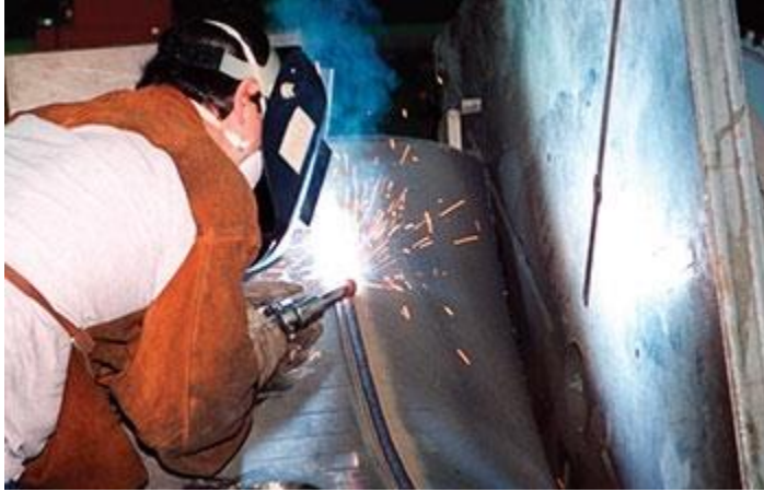
Figure 54. Flux-Cored Arc Welding (Flux-Cored)
